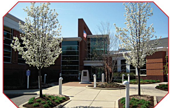
Salem Community Center
